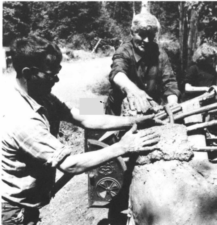
The clay blocks are laid around the arch of the doors Lise and Jean-François Blanchette Collection
