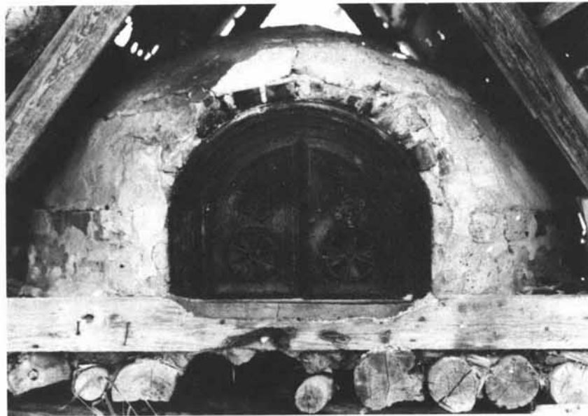
Oven built on a base of logs Saint-Honoré (Dubuc county) Blanchette Collection, NMC 73-25915
