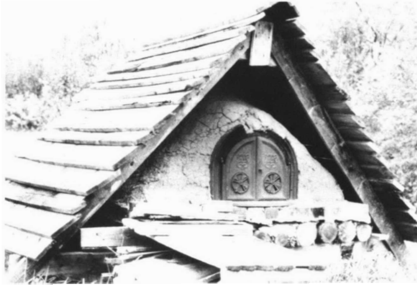
Clay oven with a clapboard roof-shelter; built at Saint-Ambroise in the summer of 1971 to commemorate the past Lac Saint-Jean Blanchette Collection, NMC AC-21-74-2
