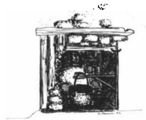
Although its dome is outdoors, the oven can be opened from inside the building by doors in the backplate of the fireplace Saint-Hilarion (Charlevoix county) Blanchette Collection, CCFCS Archives, no. 104 (interior)
