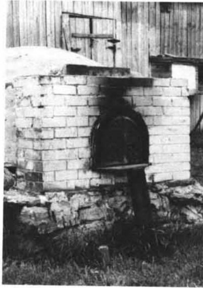
A brick wall often forms the façade of brick ovens Chambord (Roberval county) Blanchette Collection, NMC 73-25949
